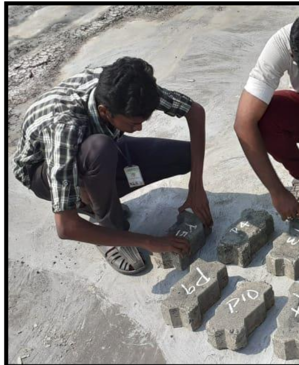
Fig: Unmolding of paver blocks
